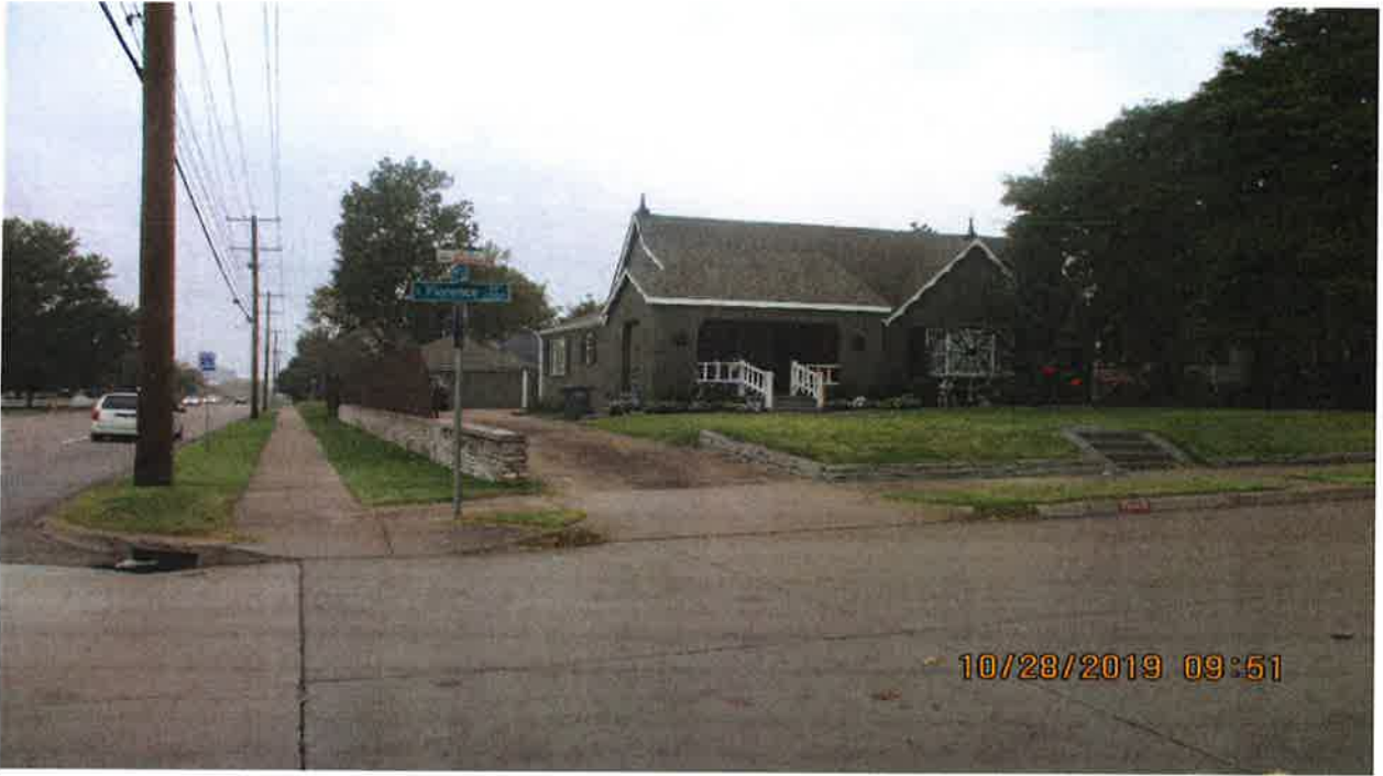
Subject property facing West
