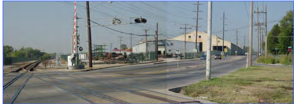
Pine Street and New Haven Avenue existing conditions looking south
