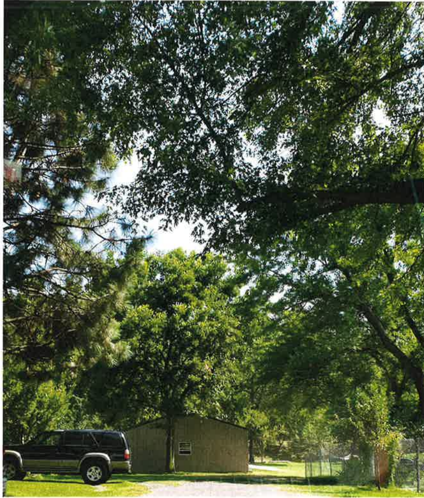
Looking south at the accessory building on the west of the property
