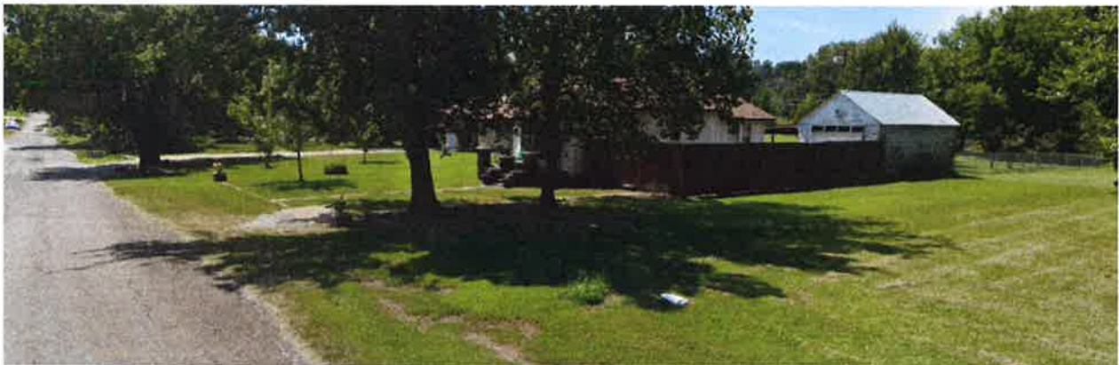
Accessory building - looking south from S. 61st W. Ave.
