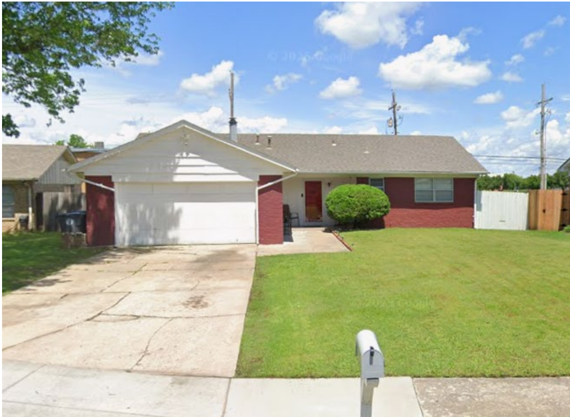
View north from East 27th Street, May 2025 (Image from Google Street View)
