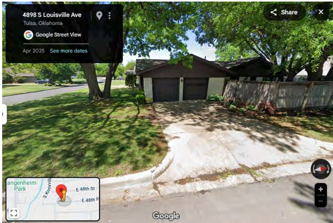
View west from Louisville Avenue, April 2025 (Image from Google Street View)
