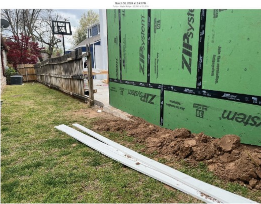
Figure 2 – With removed fence it becomes clear the ADU is not in compliance with setbacks.
