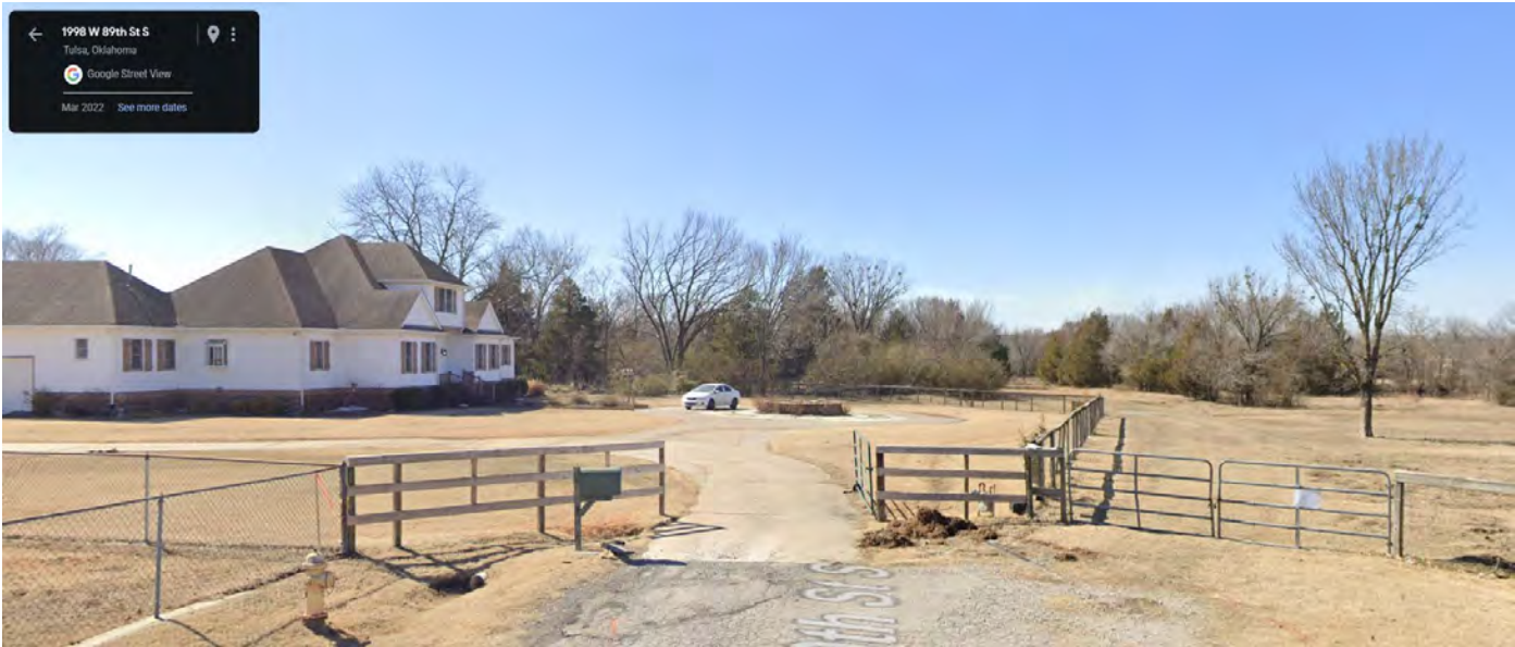
(Subject property – image taken from Google street-view)
