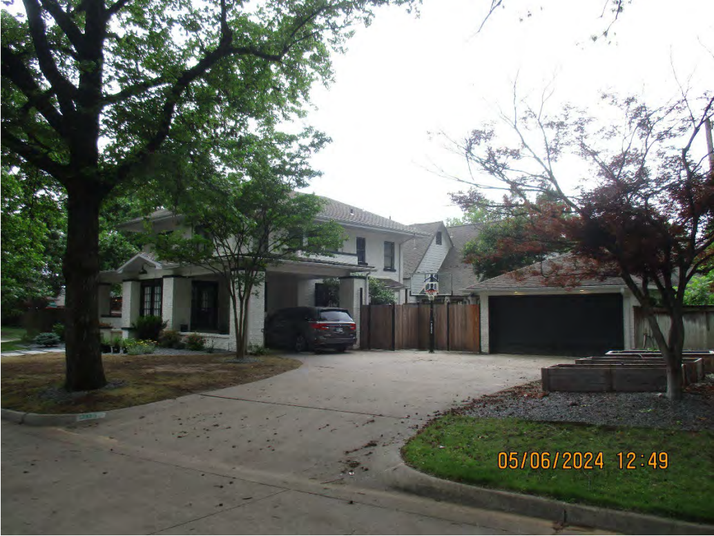
Subject property showing the residence and garage to be connected
