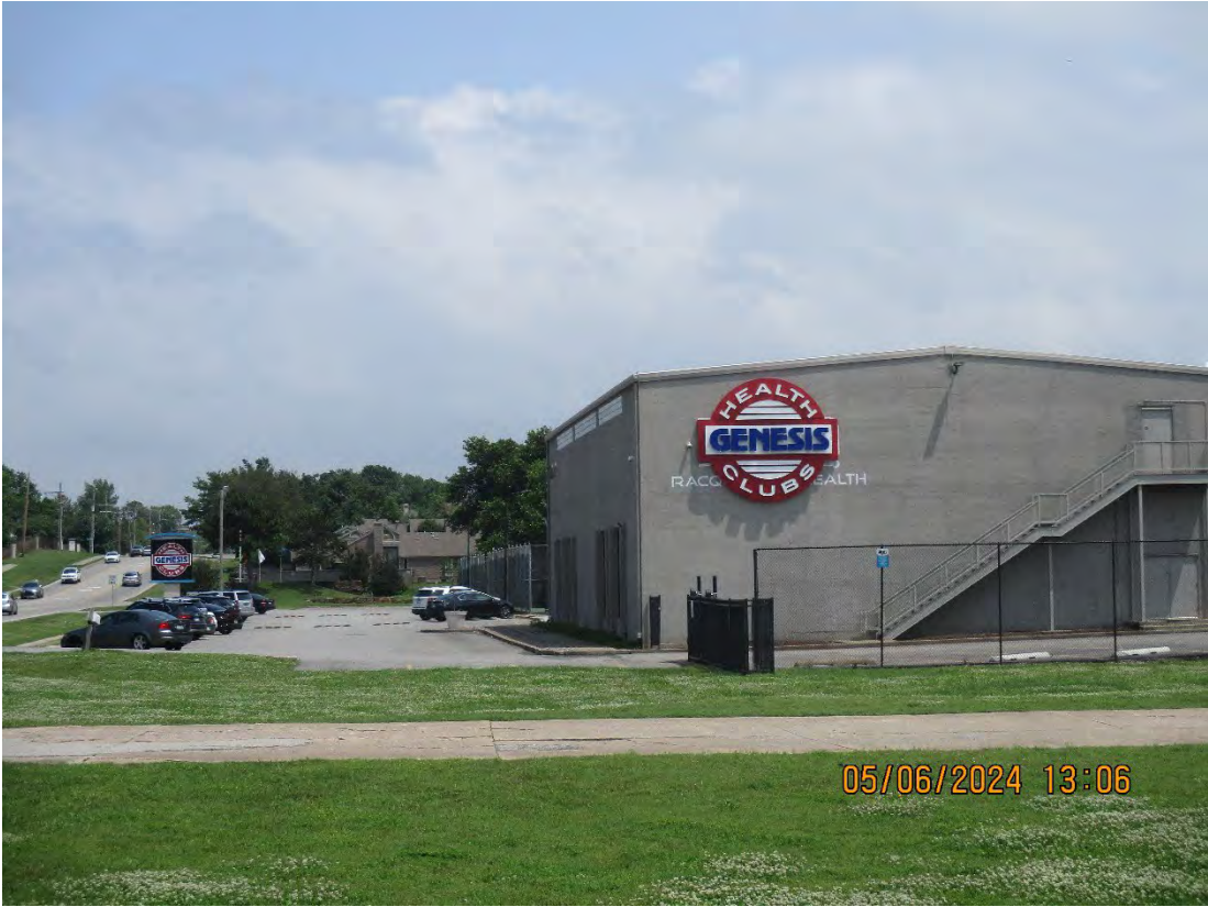
Subject property showing the subject sign that has been installed without permits
