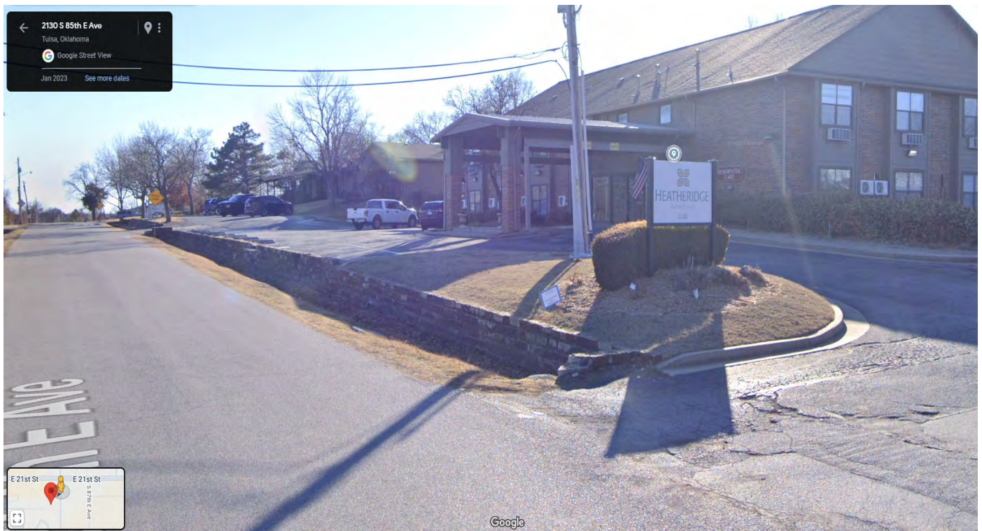
Subject property looking south on S. 85th E. Ave (Image used from Google Street view)
