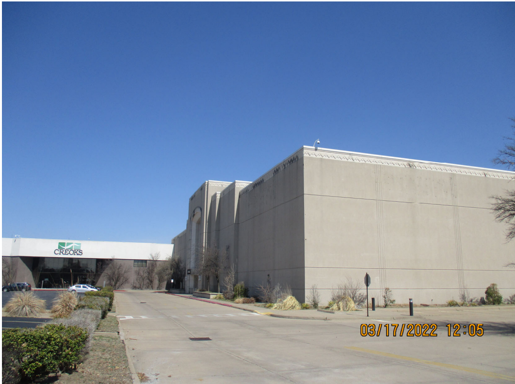
West facing Entrance of Subject property
