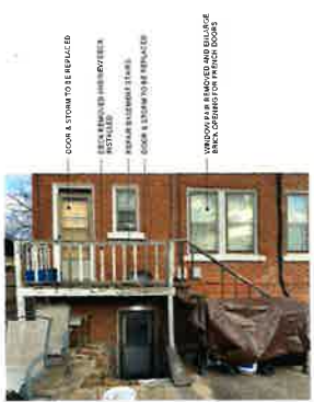
MAIN HOUSE WEST ELEVATION DETAIL
