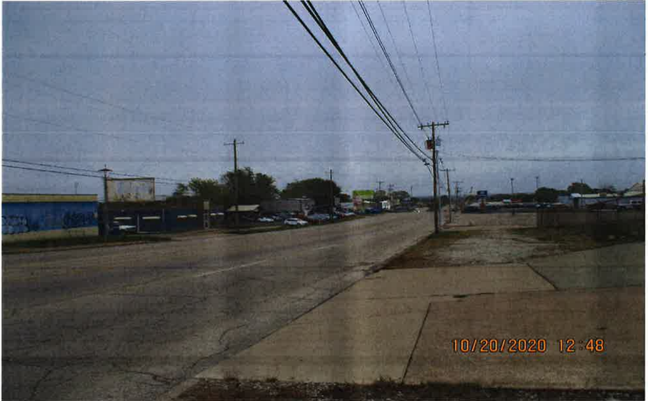
Facing East on 11 th Street
