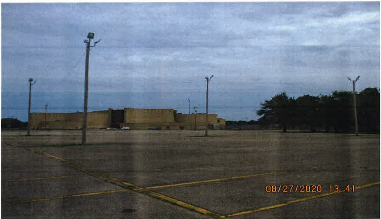
Existing School Property
