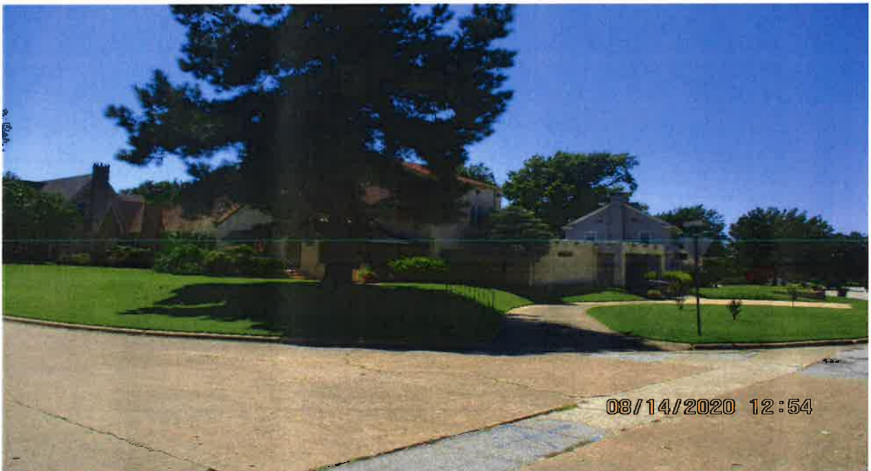
Subject property with existing Carport
