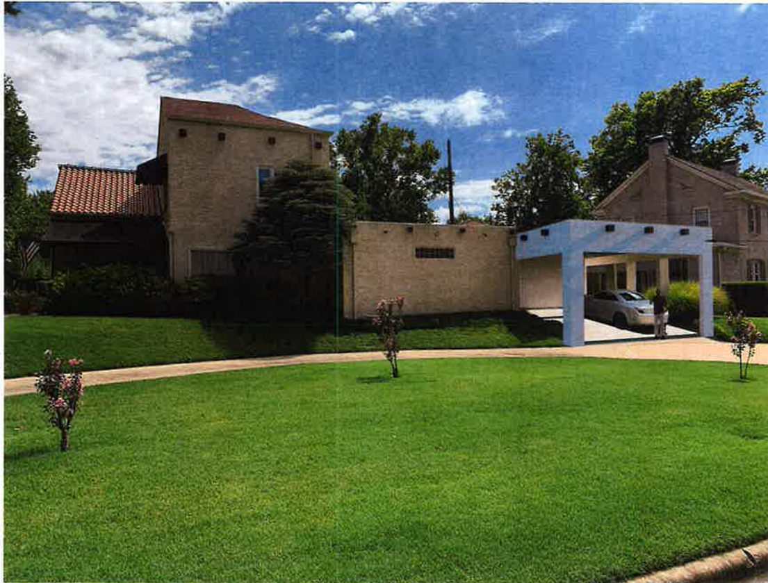
NEW CARPORT EXTENSION COLOR TO MATCH EXISTING (SHOWN IN WHITE FOR CLARITY)
