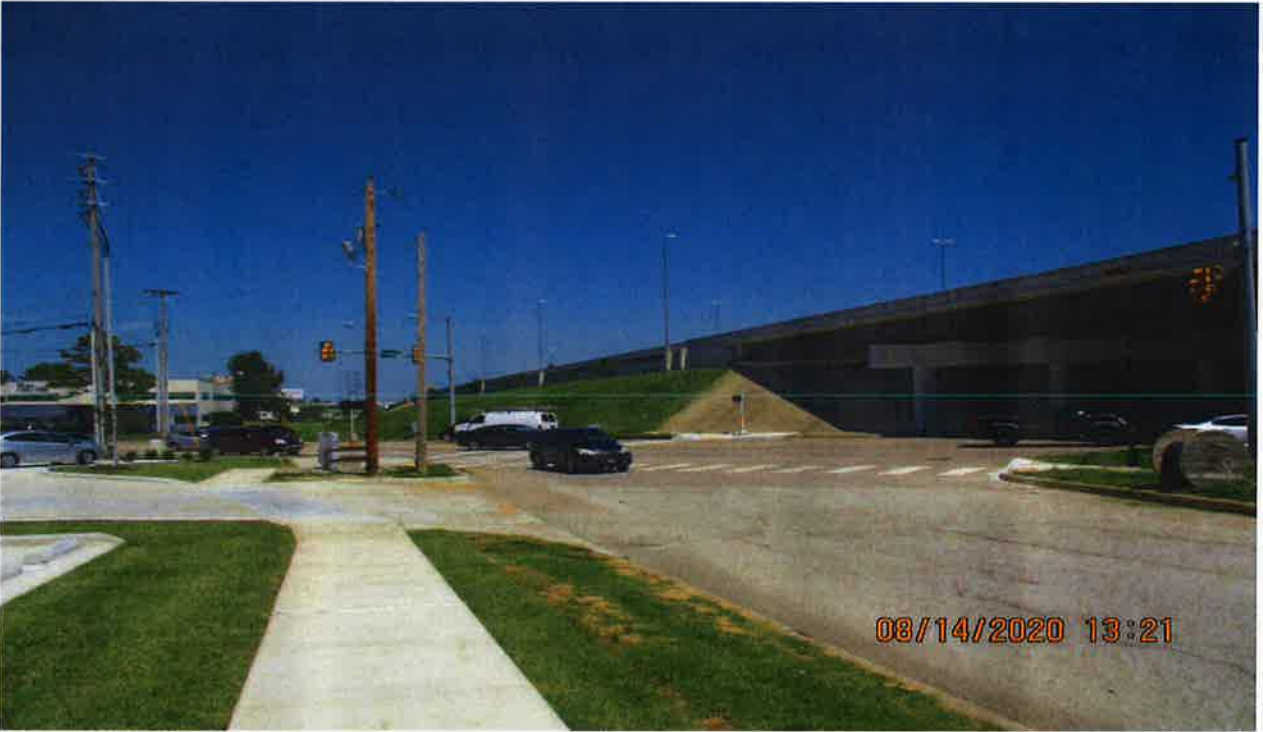
Intersection of Skelly Drive and S. Sheridan Road.
