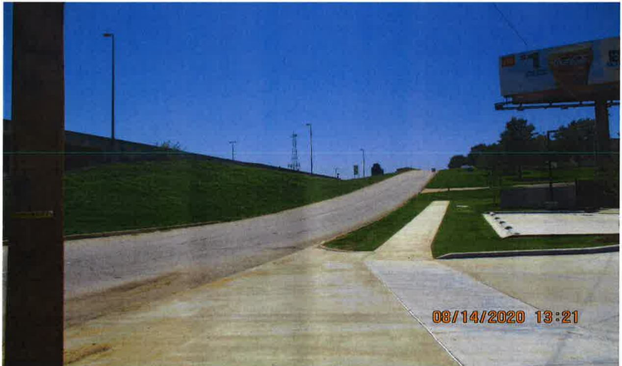
Facing West on Skelly Drive
