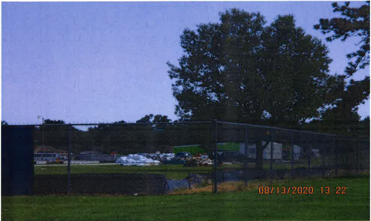
Subject property currently under construction
