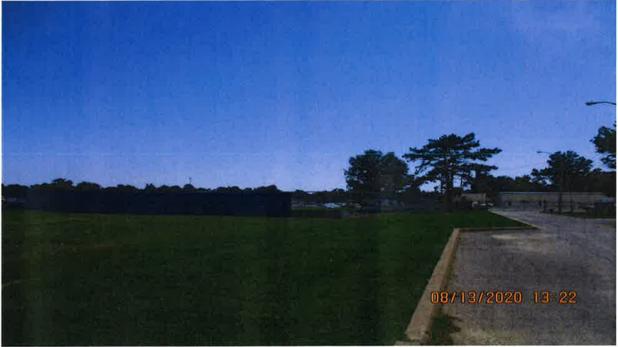
Subject property currently under construction
