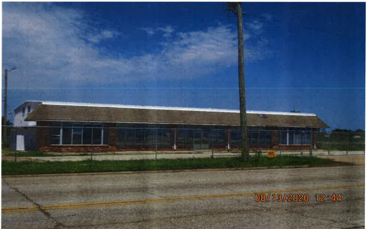
Subject property: Eastern building.
