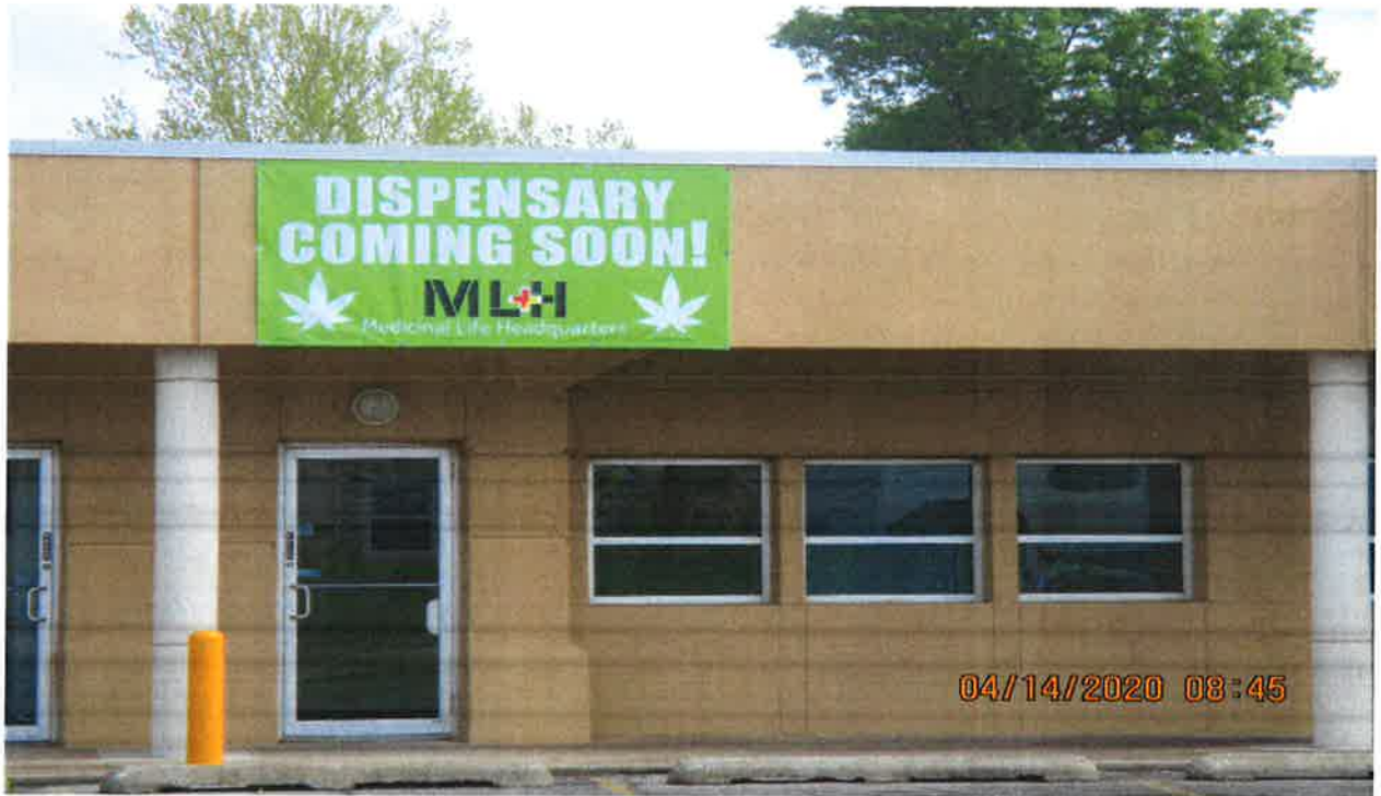
Dispensary at 6125 E. 31 st that has received their Spacing Verification in BOA-22881 and Certificate of Occupancy which is included in your packet
