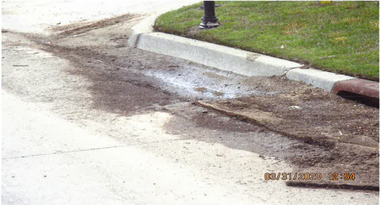
Gutter outside of business on 107 th E Ave.
