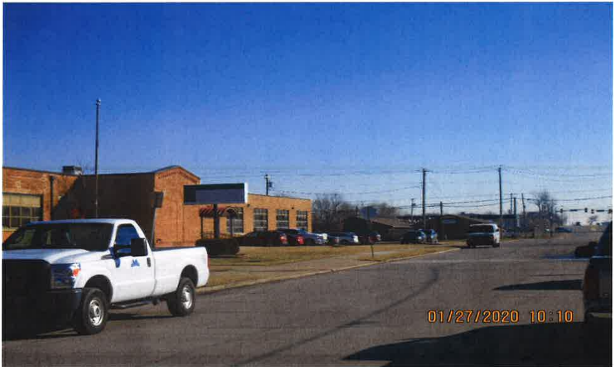
Facing East on Virgin, Tulsa MET Junior High and High School is located immediately across Virgin from subject properties
