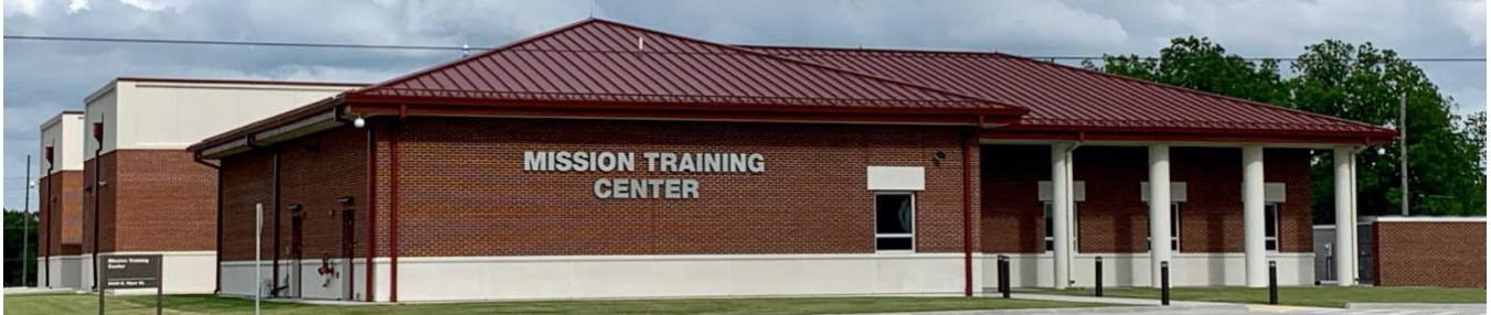
Figure 1 The newly constructed Oklahoma Air National Guard Mission Training Center
