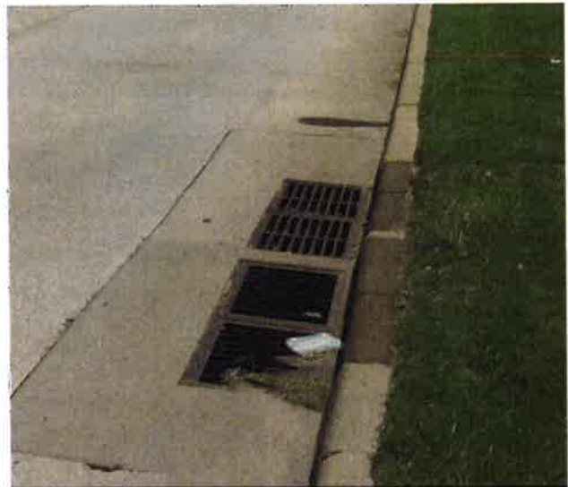
On-street facility cost estimates developed for the GO Plan include the cost of replacing storm drain grates. The region's roads today have a mix of bicycle-safe and unsafe storm drain grates. To be safe for bicyclists, the grate holes must run perpendicular to the path of travel.
