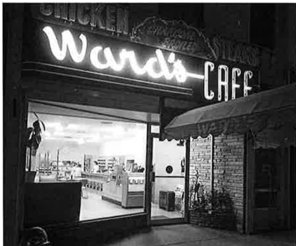
A.3.3 / A.3.5 Examples of storefronts. Important characteristics of the entries include not only the door, but the sidelights, transom windows, and display windows.
