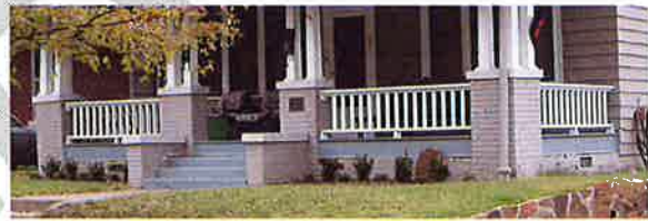
Traditional design with railing lower than piers.
