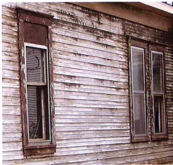
A.4.5 Inappropriate resizing (left window)
