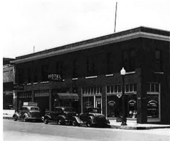
A.3.3 / A.3.5 Examples of storefronts. Important characteristics of the entries include not only the door, but the sidelights, transom windows, and display windows.
