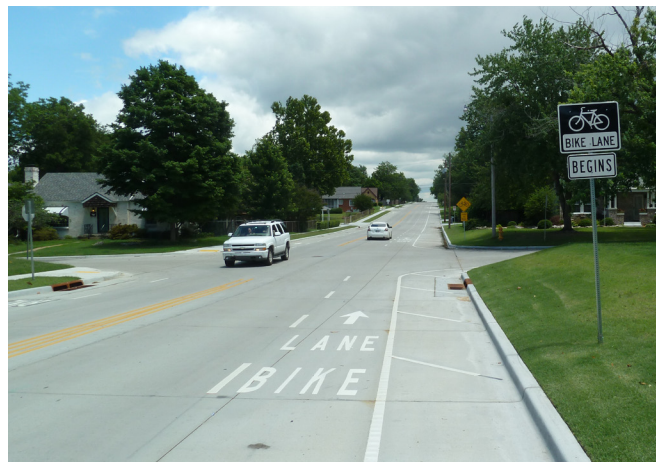
Bike lanes on 4th Place were installed through reducing automobile travel lanes from four to three.
