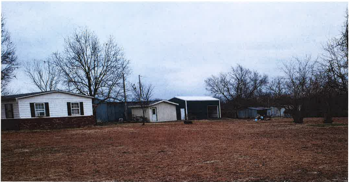
Looking northeast from N. 143 rd E. Ave. toward location of the existing and proposed shops
