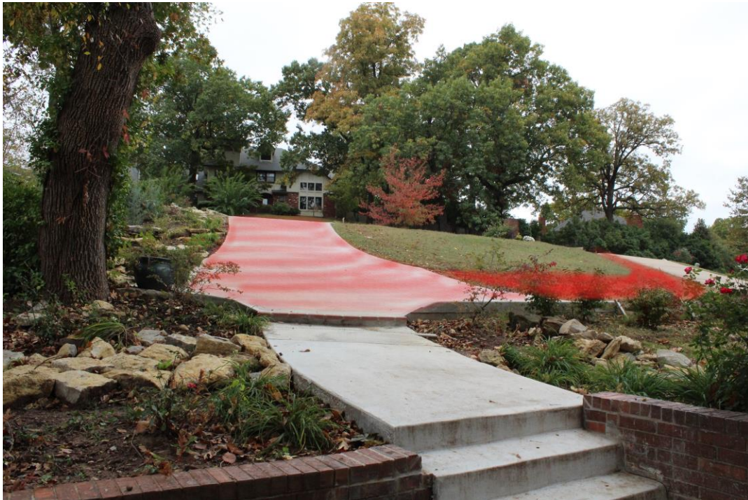
Photos of our current driveway with proposed additions in dark and light red (light red areas were poured before the project was halted). These photos show views from the house level looking up towards the street and from the street looking down toward the house.
