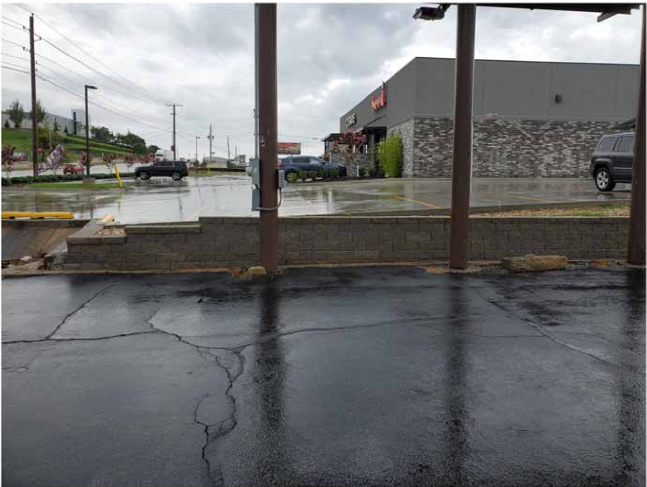
West end of the retaining wall, looking north
