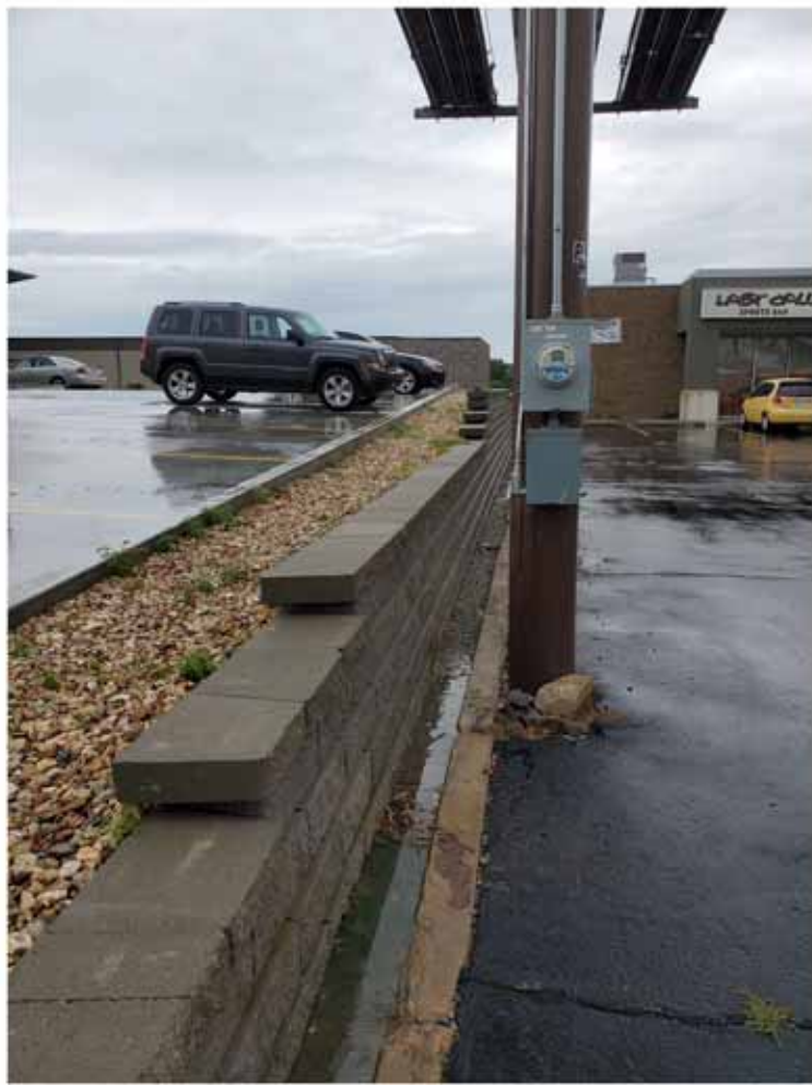
West end of retaining wall, looking due east
