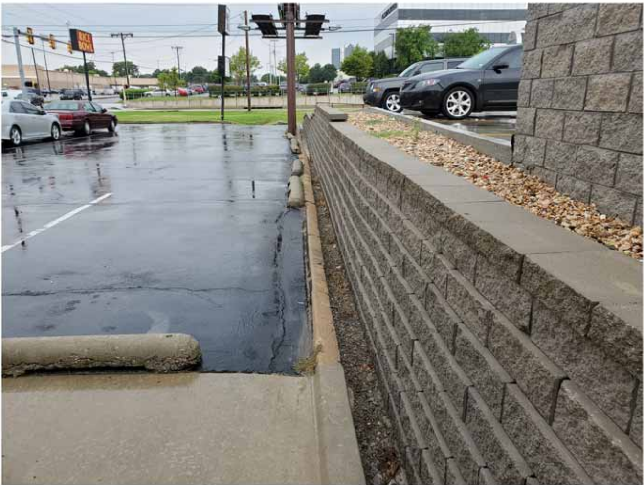
Retaining wall, looking due west.
