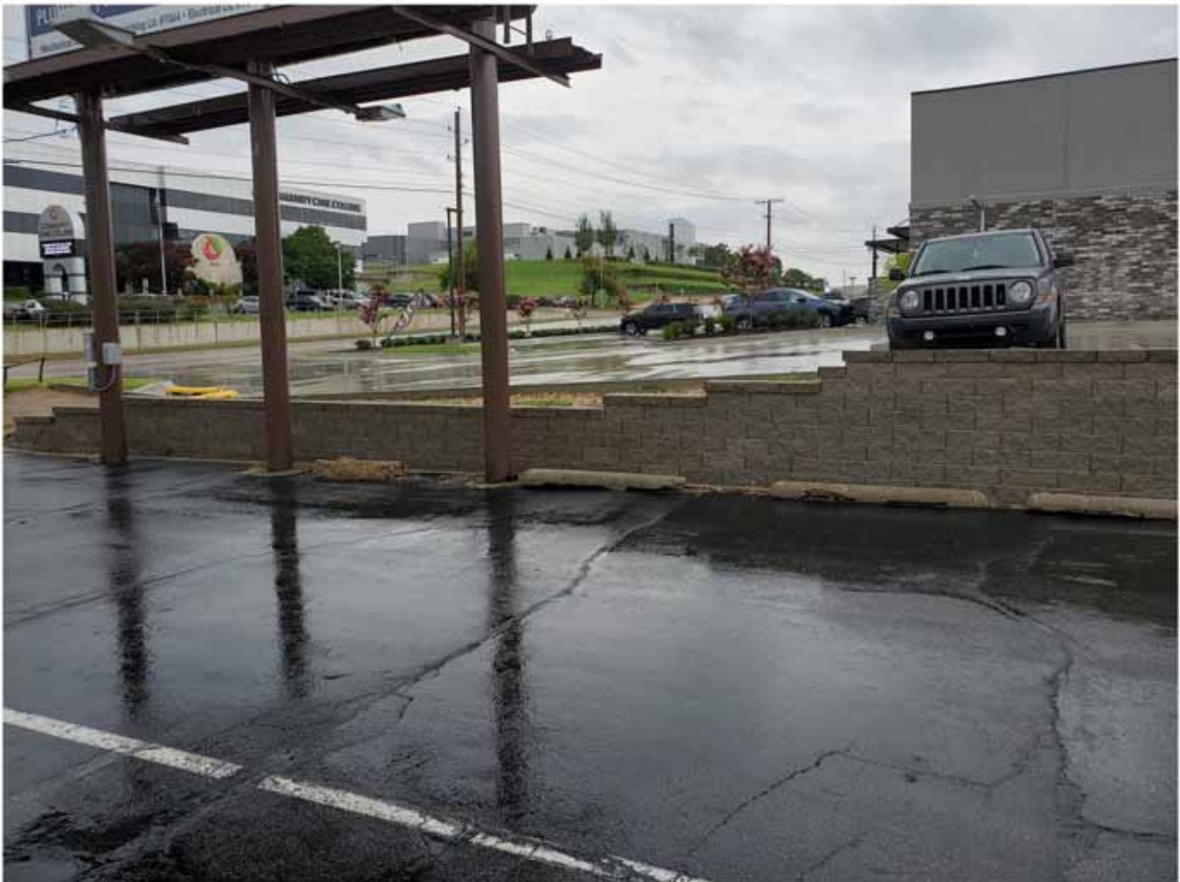
West end of the retaining wall, looking NNW
