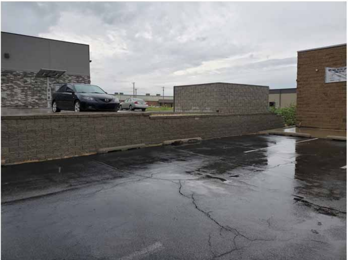
East end of the retaining wall, looking NE
