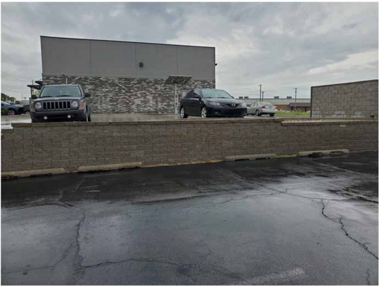
Retaining wall, looking NNE
