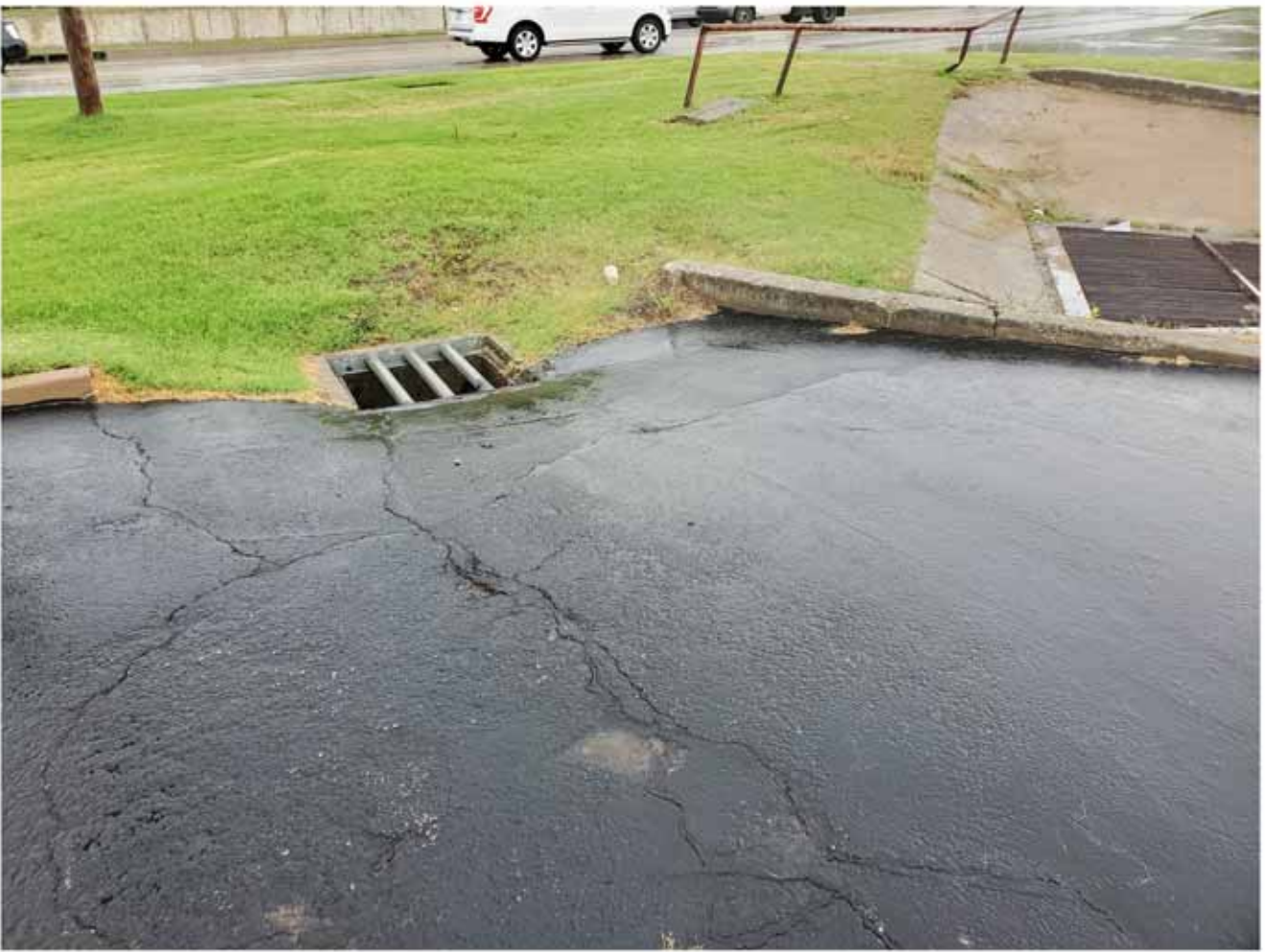
A drain at the N.W corner of the parking lot at Last Call
