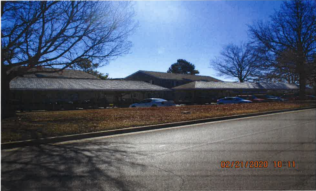
Photo of portion of the existing carports
