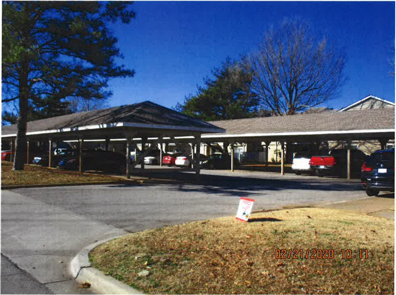
Photo of portion of the existing carports
